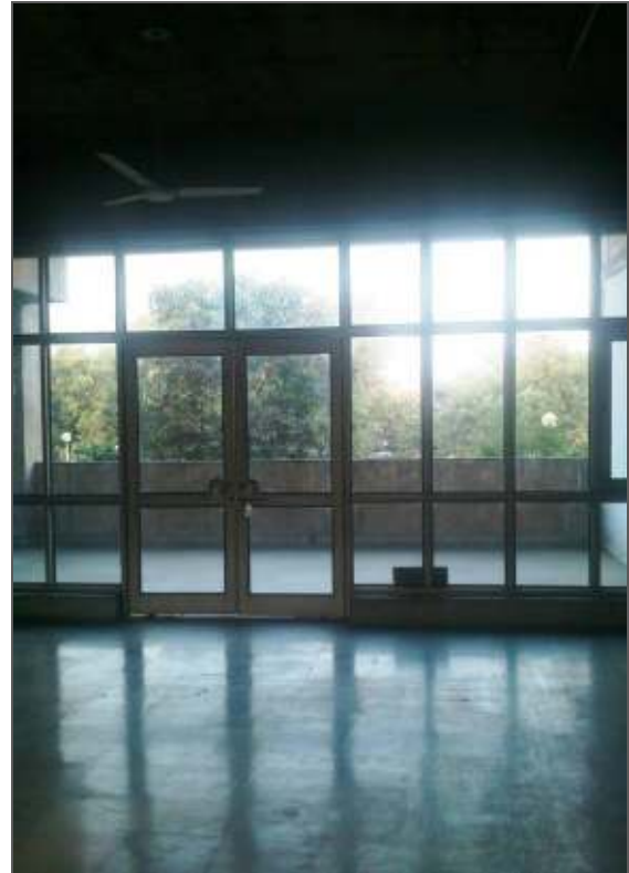
Fig 2.9 Picture: Doors complete covered by glass Panes
