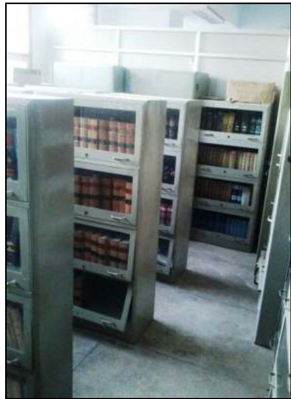
Fig 2.5: Unfixed almirahs in Library that can topple down during any disaster.
