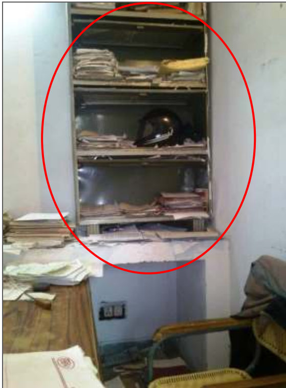
Fig 2.7 Picture showing unfixed almiahs that can topple down
