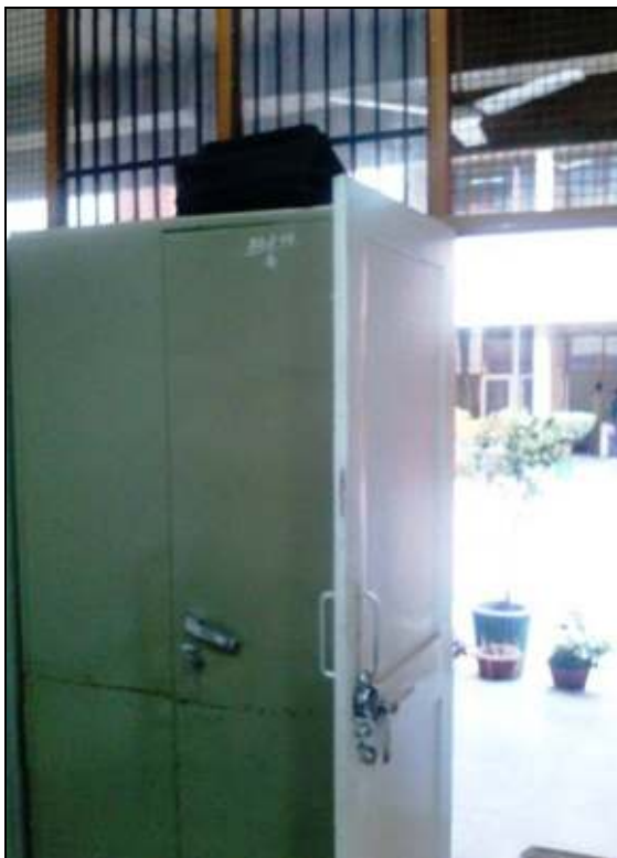
Fig 2.3: Cupboard near door capable of blocking exit
